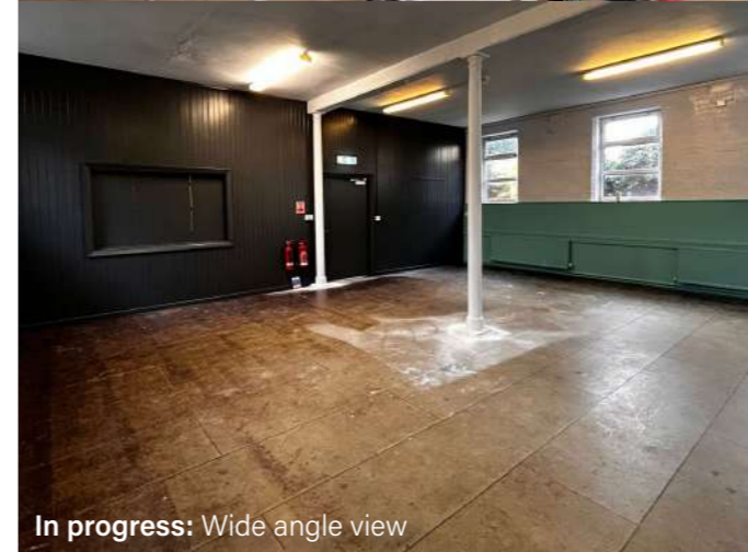
In progress: Far walls done
