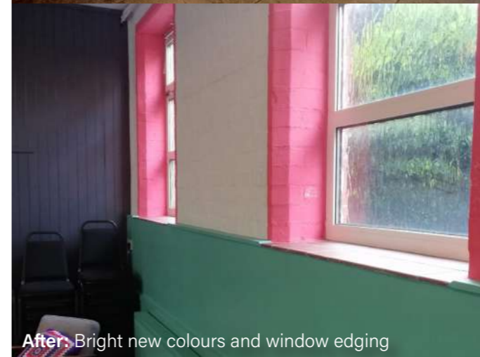
In progress: Wide angle view
